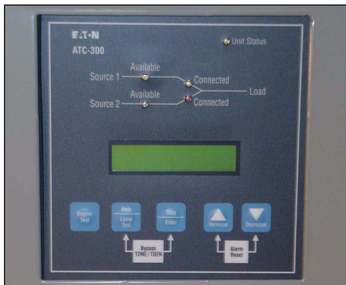
Figure 1. The ATC-300 Controller Front Panel.
